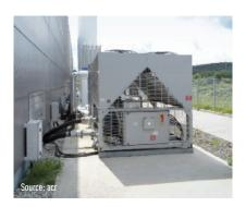
the Munich-based acr chiller rent GmbH, during the exceptionally warm summer periods of the past two years provided a constant cooling of the water in the breeding pool of approx. 28 to 24° Celsius. The water exchange rate in the four 1,700 cubic meters basins has a minimal value of only one
