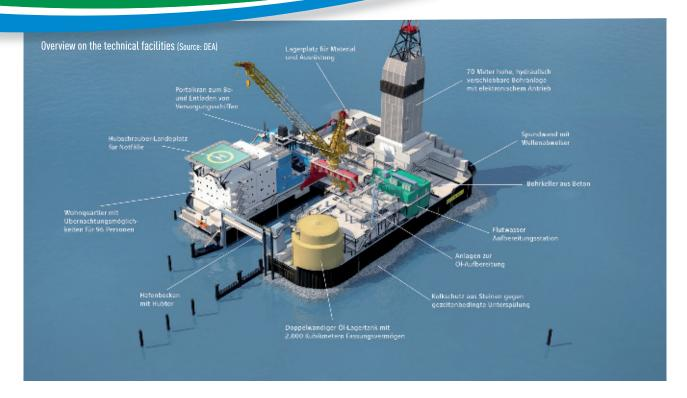
The additional cooling capacity was needed to cool the turbine during the well regeneration phase. The methane gas released during the oil recovery process is burned and used to generate energy. The use of methane as an eco-friendly additional energy source plays a particularly important role in the demanding environmental concept of Mittelplate.
